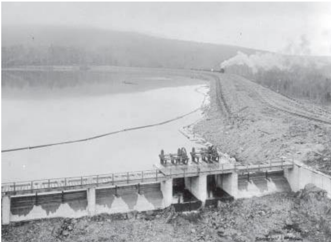
Somerset Development, built 1911-1913. View of 2,100-foot, 110-foot high modified earth fill dam looking south with spillway in foreground.
