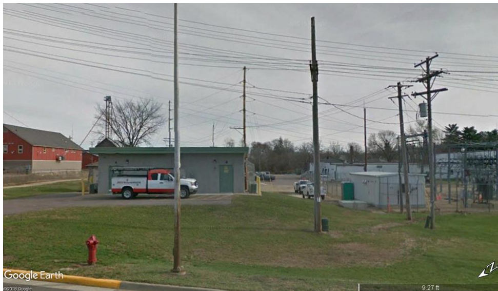
Figure 6-21: Electrical and telephone switching stations in Reedsburg, Wisconsin. The old one is to the right with the green cabinet next to it; the new one is to the left, behind the pickup truck.
