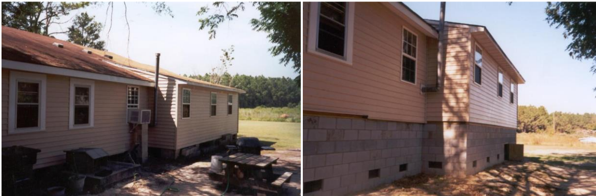
Figure 2-33: Before (left) and after (right) elevation photos for a single-family house (Source: Stacy Wright)
