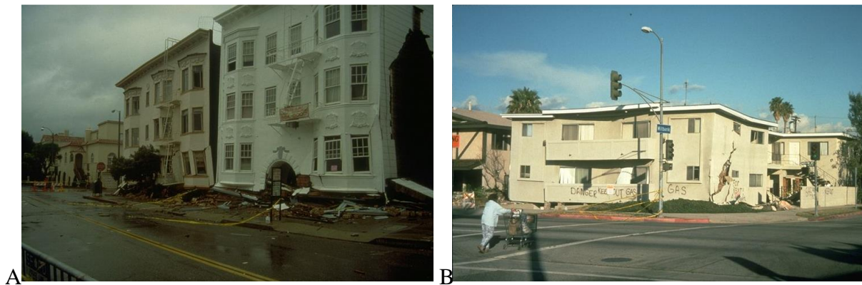
Figure 2-50: Examples of collapsed soft-story wood-frame multifamily dwellings. (A) Collapsed apartment buildings in the San Francisco Marina District after the 1989 Loma Prieta earthquake (Image credit: R.B. Seed, 1989, via UC Berkeley NISEE, with permission). (B) Apartment building collapse after 1994 Northridge earthquake, associated with soft-story conditions (Image credit: UC Berkeley NISEE, 1994, with permission).
