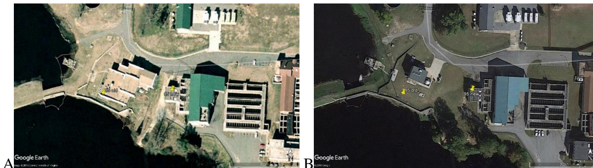
Figure 6-11: Portsmouth's water treatment plant: A) in 2003, and B) in 2015.
