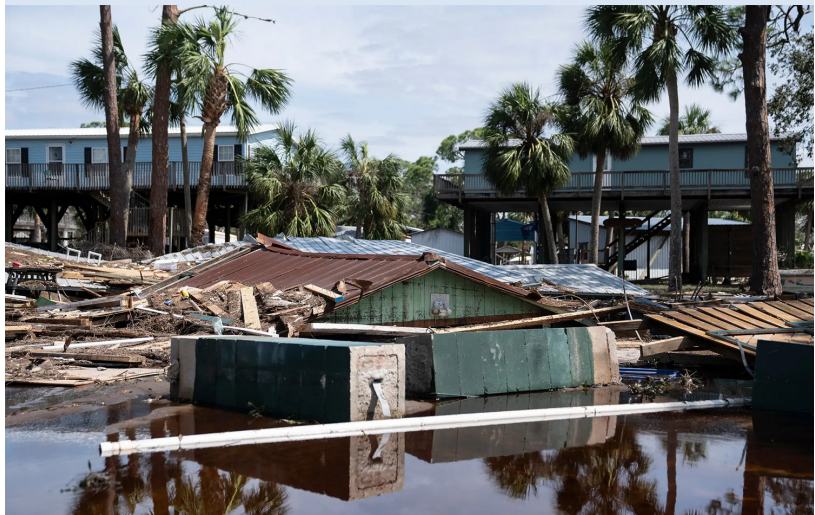
Damage from Hurricane Helene in Horseshoe Beach, FL. Photo: Nicole Craine/ New York Times .
