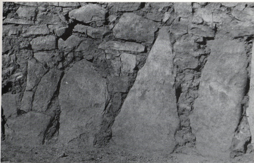
PLATE 11. Kiva A, base of banquette. Note use of vertical slabs and masonry.
