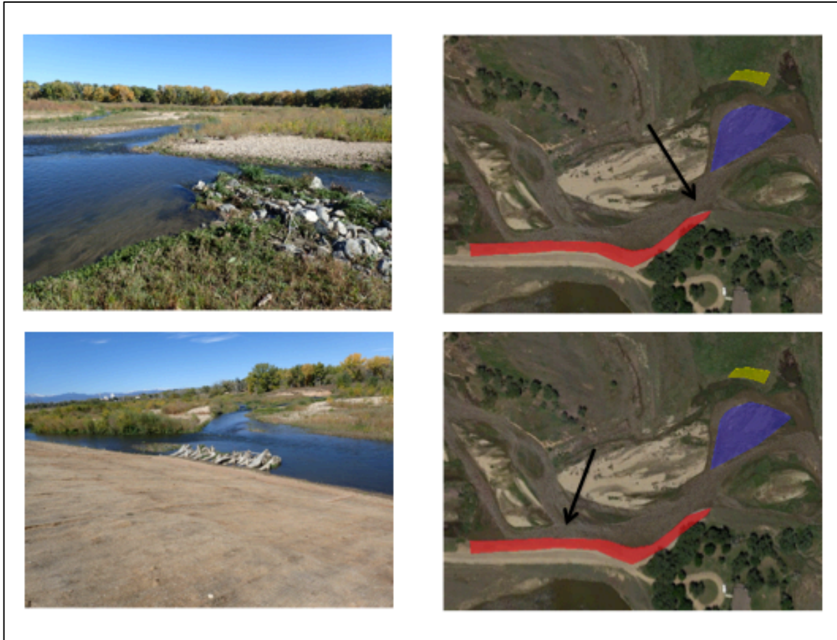
Figure 18 – Additional structures that were placed along the edge of the riprap and may have contributed to the channel diversion in the direction of the restoration site are featured on the left. Their relative position along the stream is indicated on the right by the black arrows.
