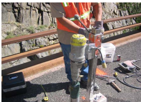
Figure 5.6 Take coring samples
