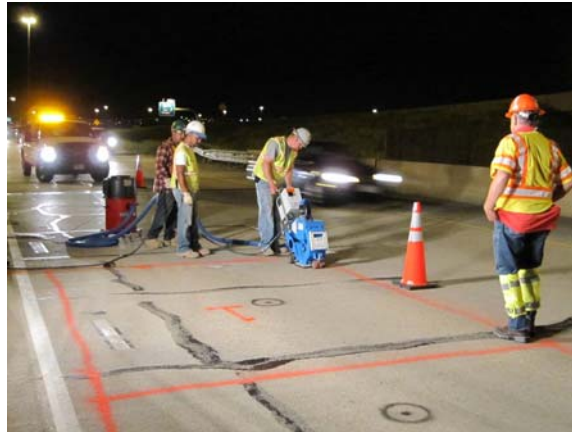
Figure 6.5 Smooth the surface
