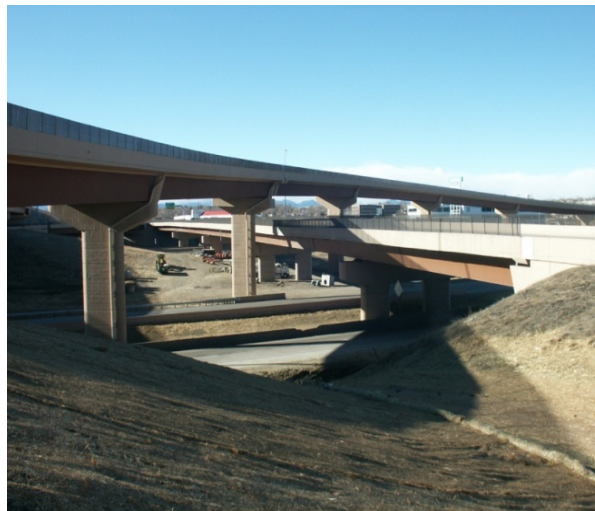
Figure 6.2 Side view of this bridge structure
