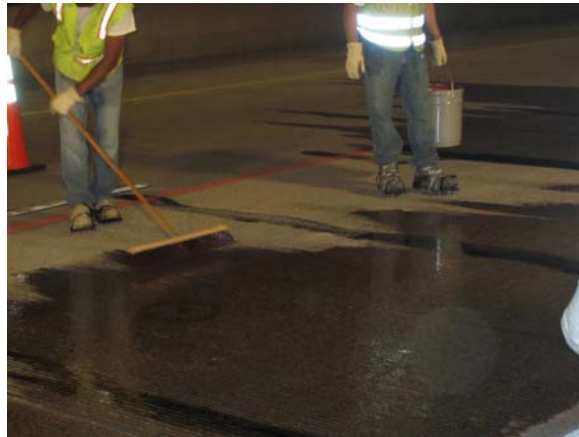
Figure 6.7 Sealer application
