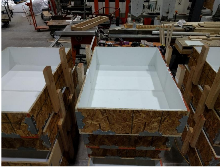
Figure 27 - Assembled and painted formwork without upper brace. Seventeen forms were built in total.
