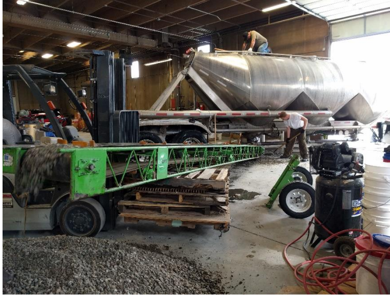
Figure 30 - Offloading aggregate
