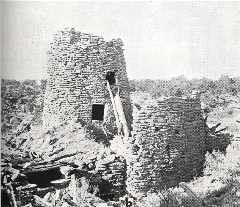
PLATE 12. Site 6. a , view from southwest; b , close-up of tower from the north.
