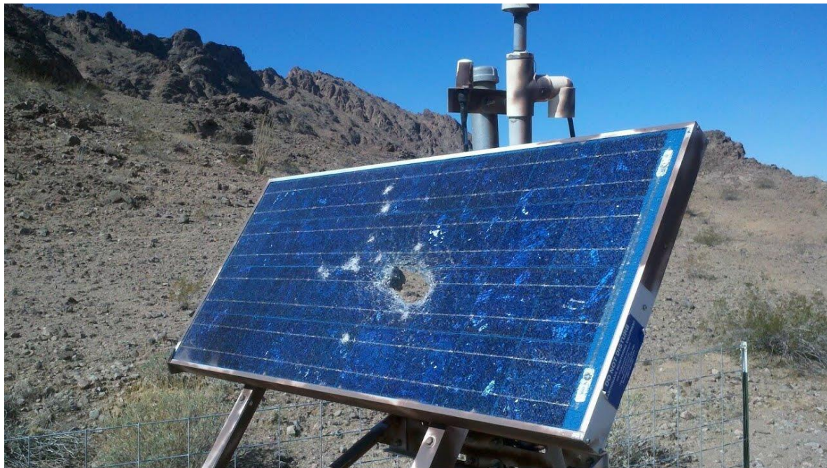
Image 1: Broken Solar Panel from Thrown Debris
