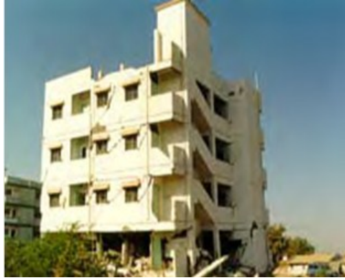
Figure 1-1. Masonry infilled frame in India (Jaiswal et al., 2002).
