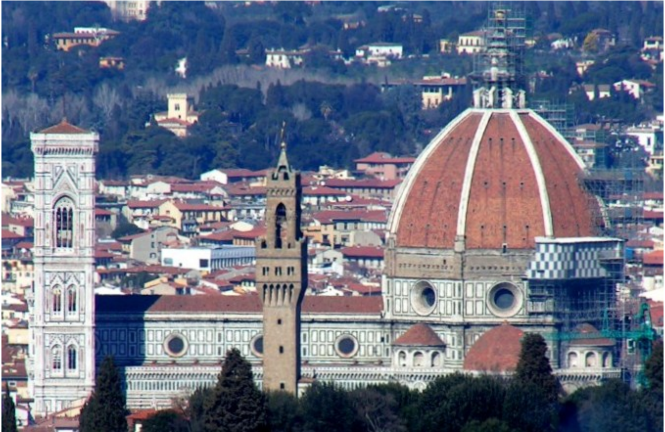
Designed by Filippo Brunelleschi and completed in 1436, Il Duomo, the dome of the Florence Cathedral, was built in the early 1400s without the aid of scaffolding..
