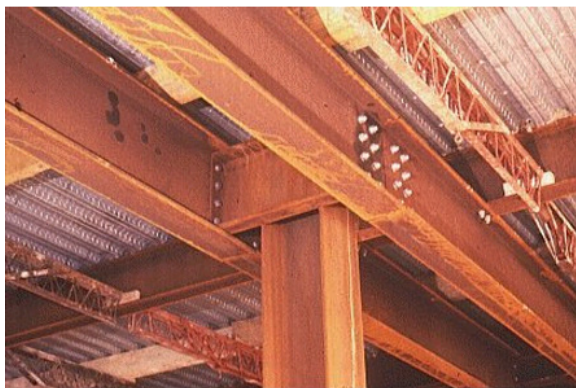
Figure 2: Web Splice (Corus Construction n.d.) & (Kulak 1975)
