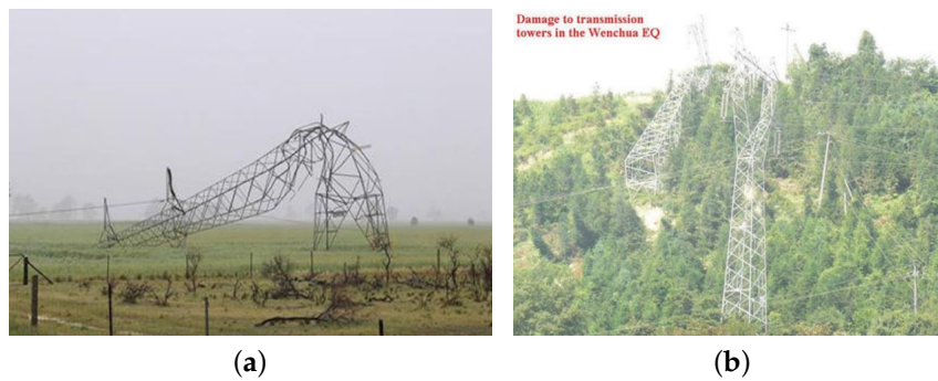
Figure 1. Potential failures in power transmission towers [2,3]. (a) Wind-induced failure; (b) Earthquake-induced failure .
