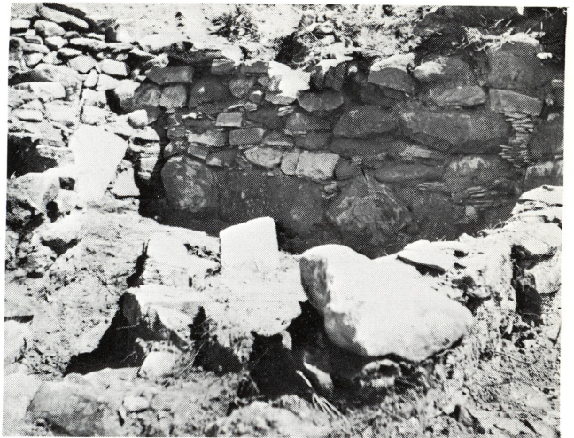
FIGURE 10. North wall of Room 12, Site 1088. Note use of large stones in lower portion of wall and potsherds as spalls between the masonry.
