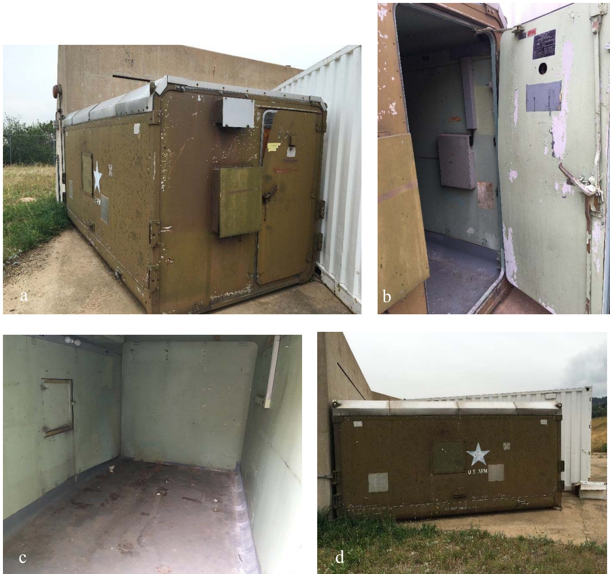
Figure 6.1. Photographs of the bunker are presented. (a) Exterior front and side of the bunker. (b) Open hatch on the front wall. (c) Bunker interior. (d) Side view of the bunker; one of the walls into which sampling ports were drilled.
