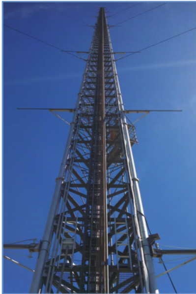
Figure 2. Photograph of the BAO tower, looking up at the southwest face. The northwest booms are pictured extended to the left, with the southeast booms to the right. The elevator and carriage tracks are pictured in the center of the southwest face.
