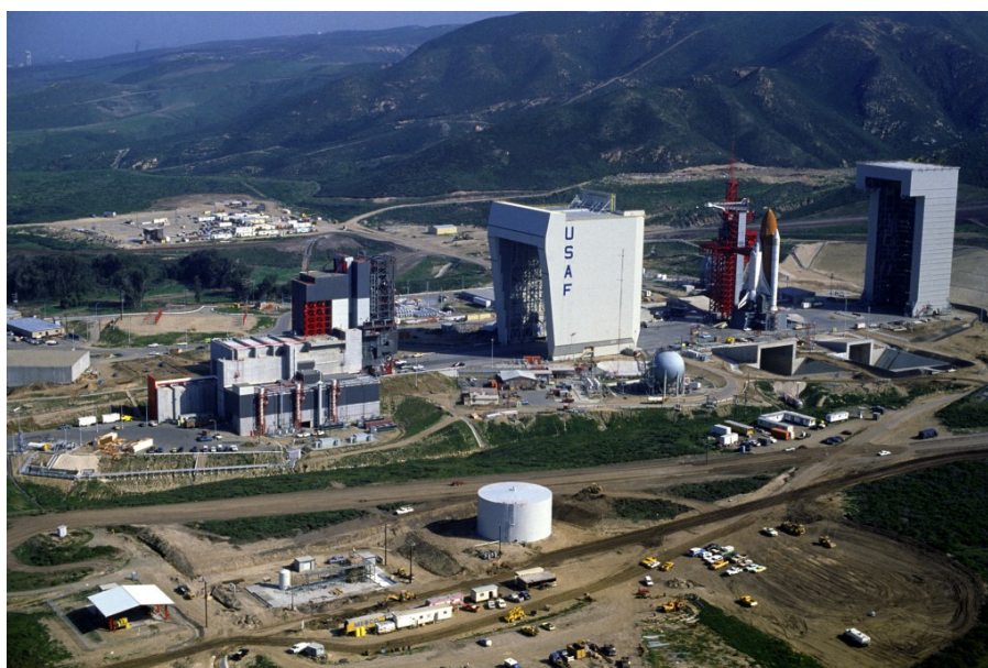
Figure 5.3. The SLC-6 “Slick Six” launch complex at Vandenberg AFB, with the Enterprise test orbiter in a launch configuration mockup. Source: U.S. Air Force.
