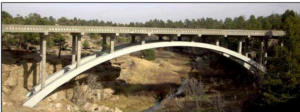
Figure 2. Castlewood Canyon bridge, Franktown, Colorado.
