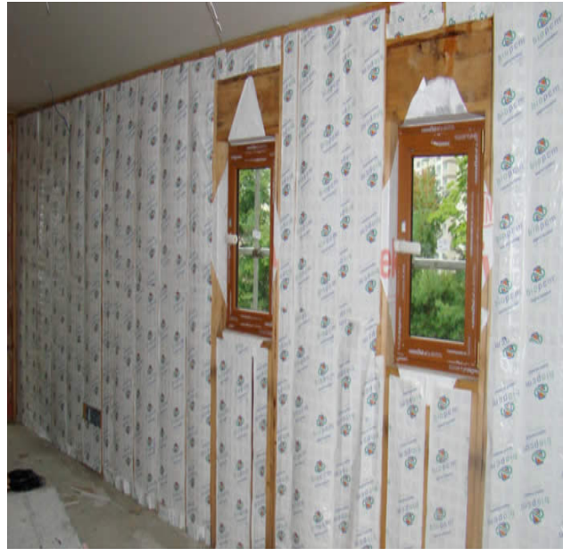
a) BioPCM® Matt by Phase Change Energy Solutions [272] b) BioPCM integrated into wall systems [272]
