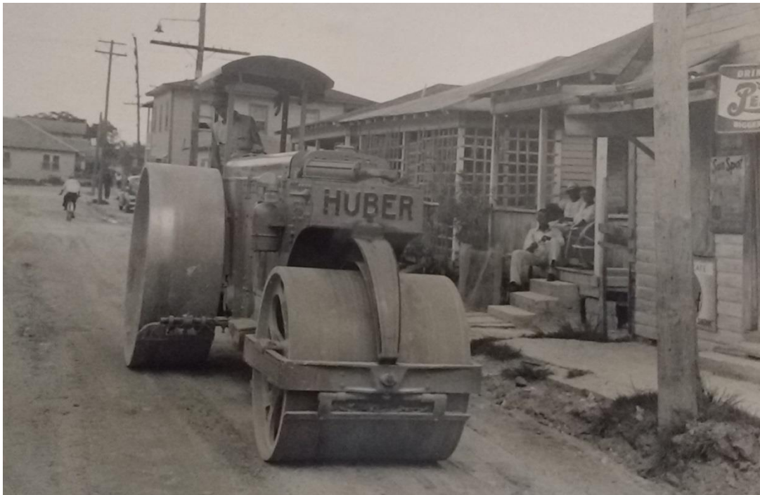
A Huber 10-ton diesel roller on a newly graded Miami street, 1941. Aesthetically, the machine remained almost unchanged since Gifford first designed it in 1923; Gifford Papers
