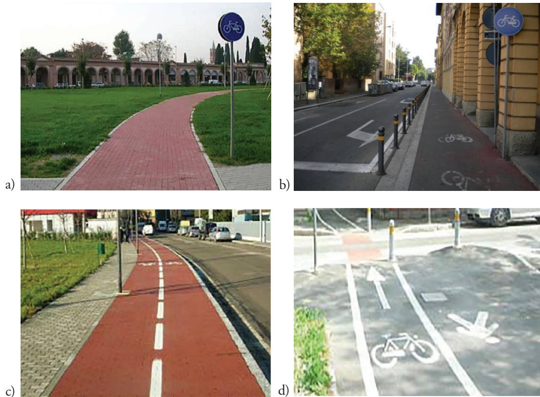
Figure 1: Some examples of the off-street facility typologies in Italy, as categorized in the Italian regulation: a) separated path non-adjoining the roadway; b) separated path, separation obtained by a non-continuous barrier; c) cycle track, obtained from the sidewalk, separating pedestrian and bicycle areas with different pavements; d) cycle track, obtained from the sidewalk, separating pedestrian and bicycle areas by painted markings.
