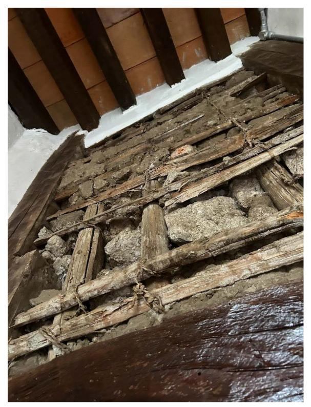
Figure 4.7 Interior open wall inside friars' quarters at San Miguel el arcángel, Huejotzingo featuring indigenous construction technique, 16th century. Photograph by Lauren Hooten 2023.
