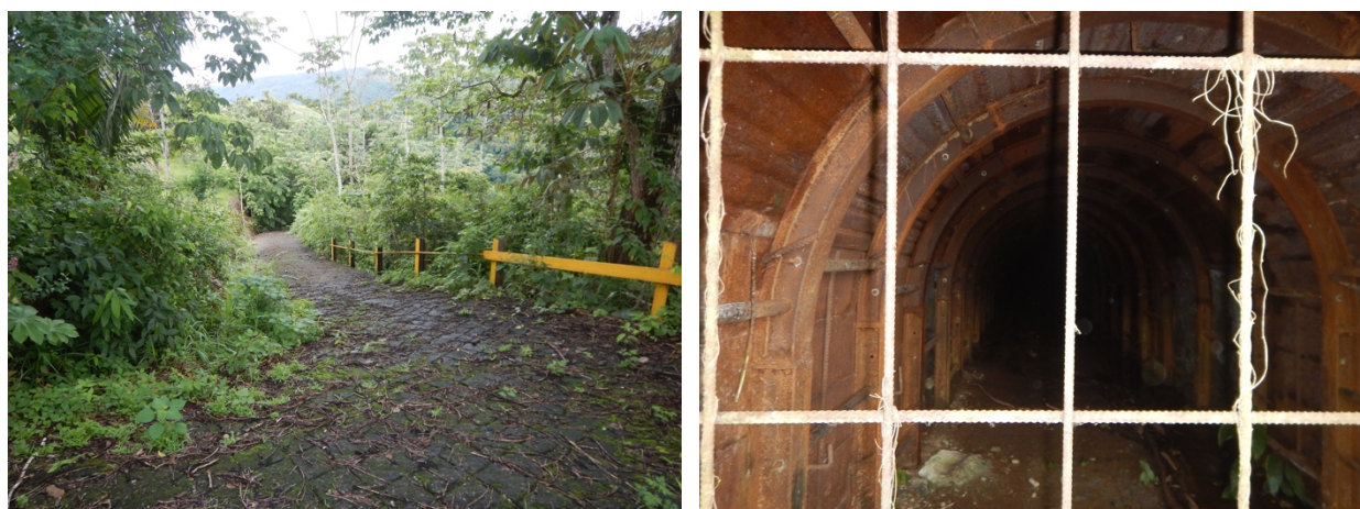
Figure 7. Left (a): Overgrown, mossy, cement road to the proposed Diquís dam site. Right (b): A look inside the first tunnel, with its rusty arched ceiling. The front was blocked by metal rebar gates visible in the foreground.
