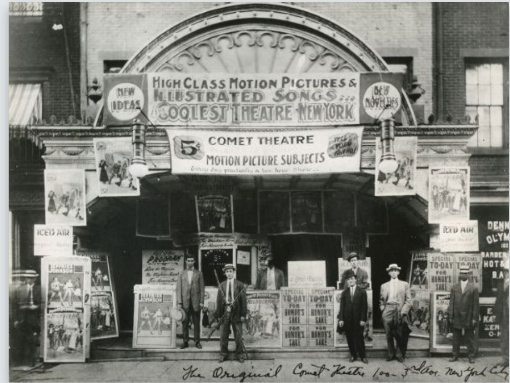
Comet Theatre, 100 3rd Avenue, New York City (ca. 1915)
