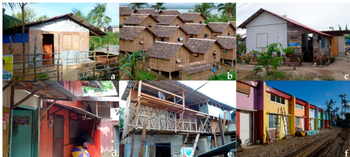
Figure 2. Example Shelter Typologies: (a) repair and retrofit; (b) transitional shelter; (c) core/progressive shelter; (d) rental subsidies; (e) hosting support; (f) resettlement.
