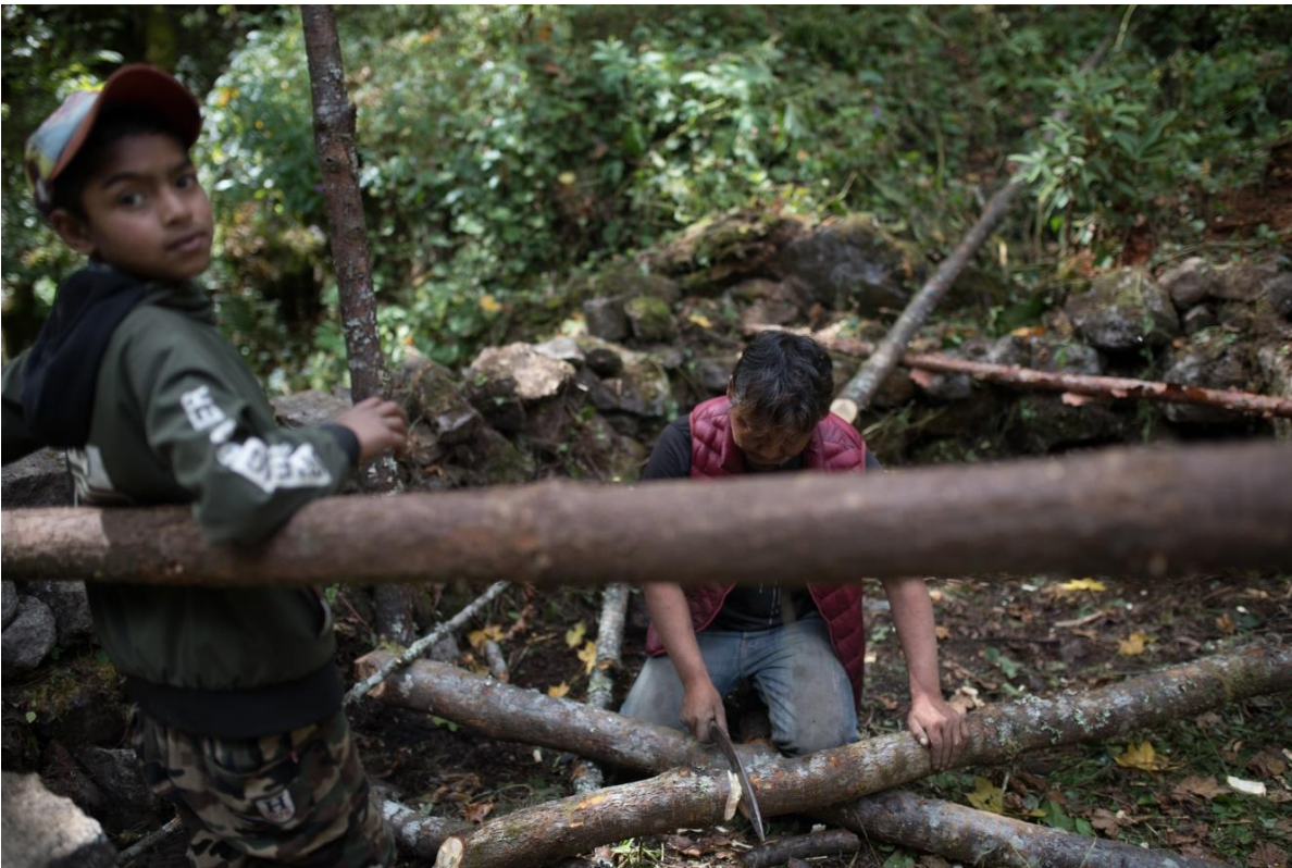
Tashi constructing a teashop along the trekking trail in Phale
