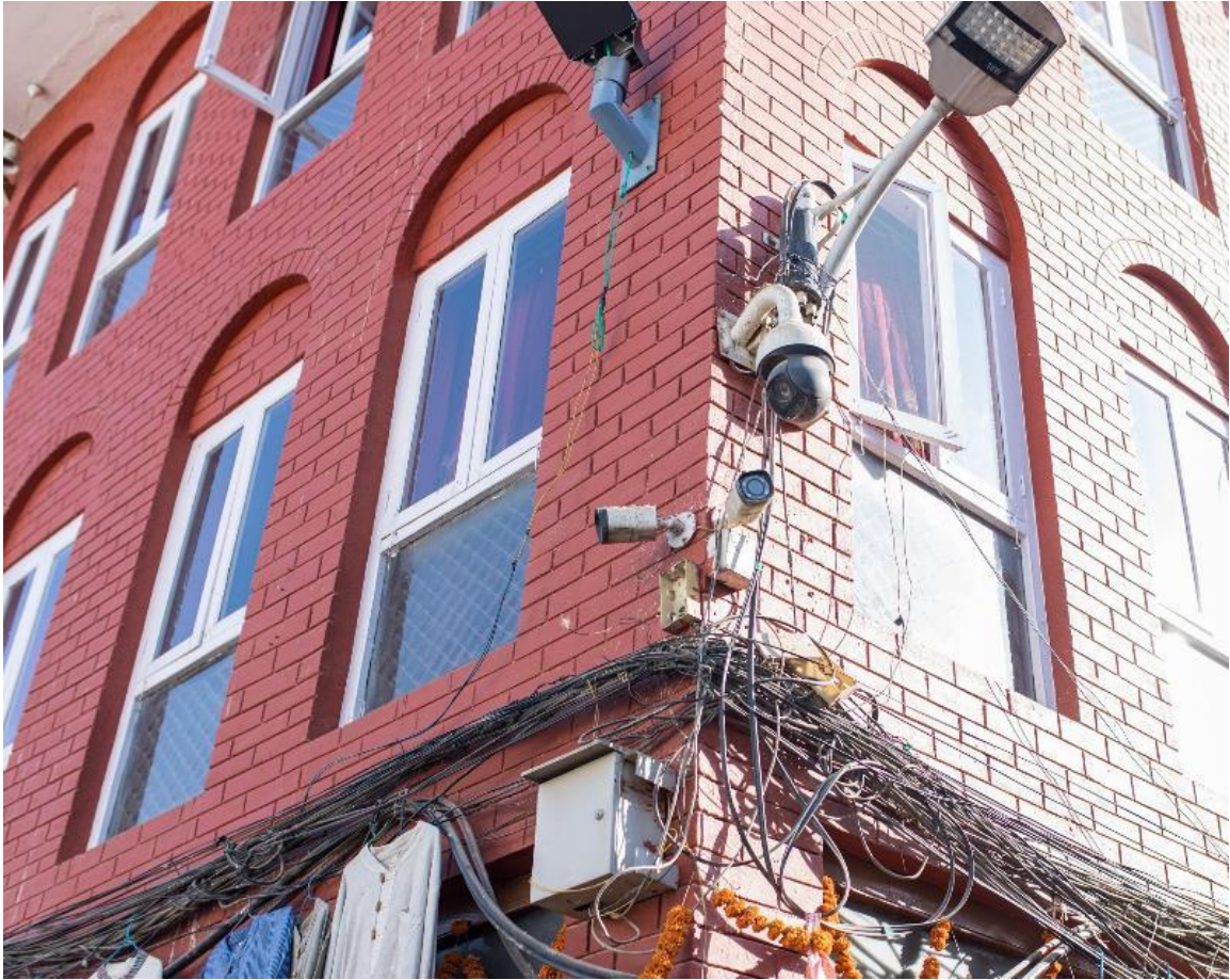
Figure 3.2 CCTV cameras at the eastern gate of Boudha.
