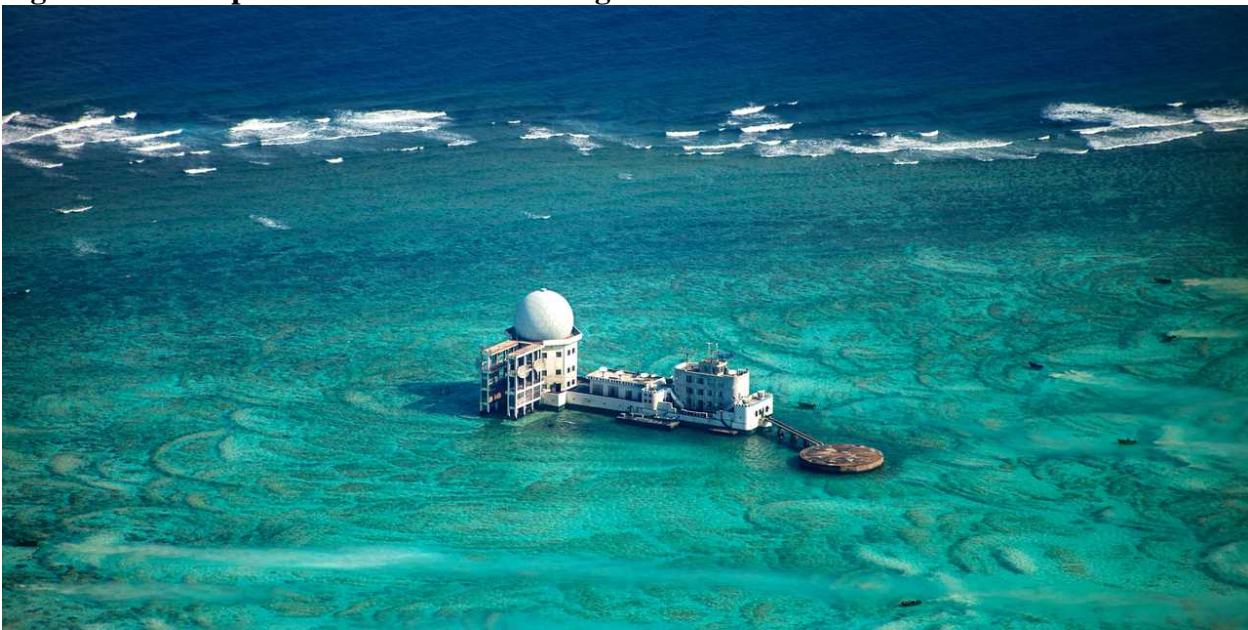
Figure 80: Example of a Pre-Island-Building Structure on Subi Reef
