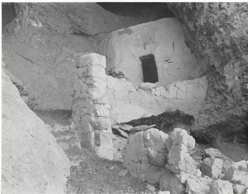
B. Zigzag Cave. Walls shown are constructed of puddled adobe mud with a few unshaped stones incorporated.
