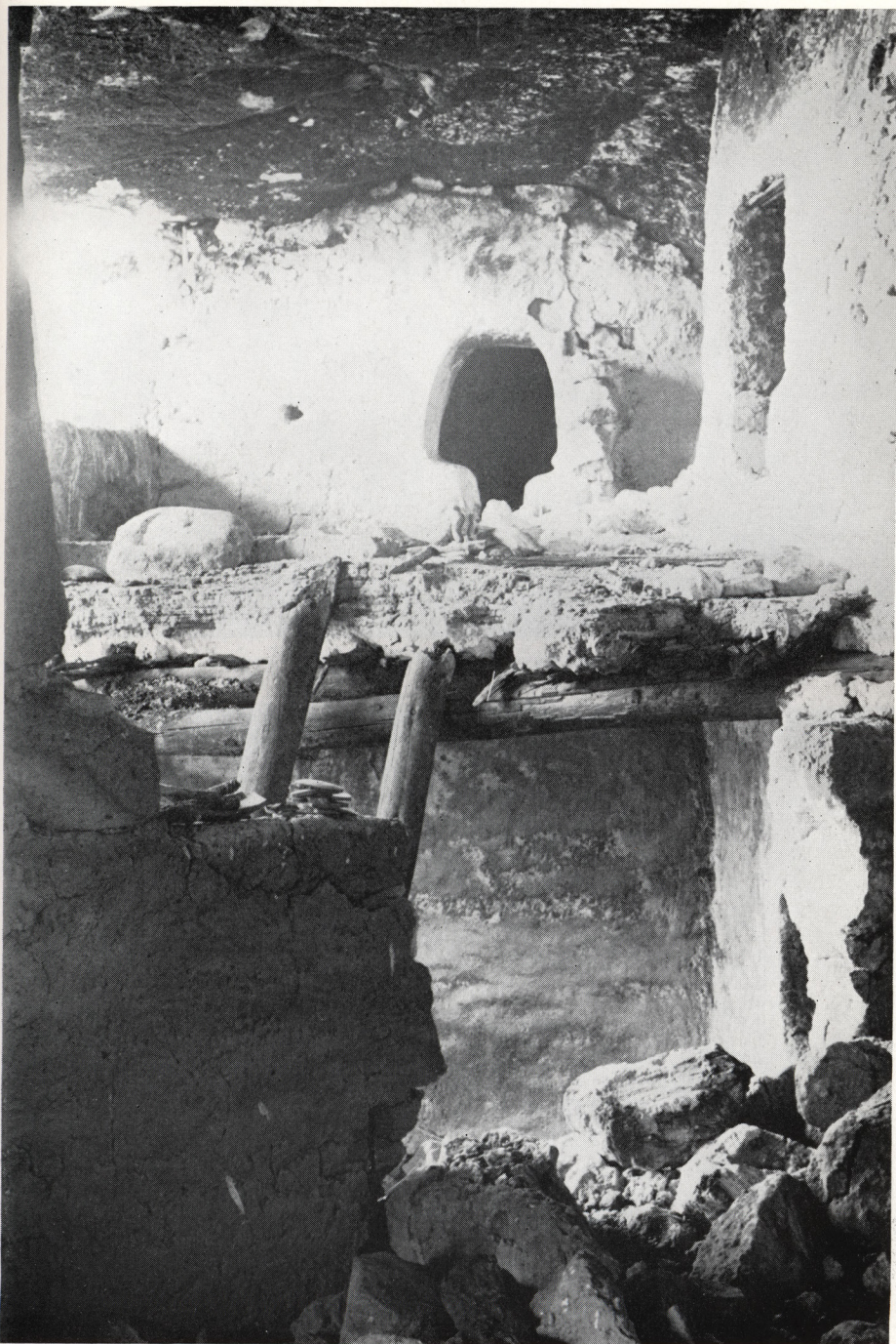
Step Cave, Arroyo el Concho, Sonora. Method of roof construction is shown
