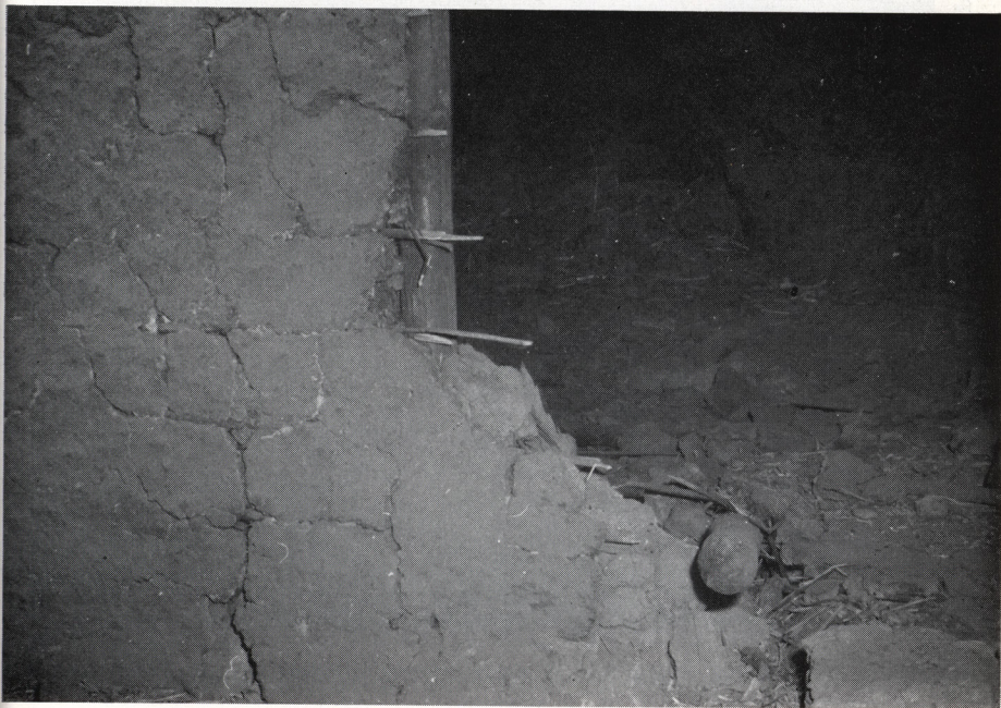
B. Corral Cave. Portion of a post-and-mud wall showing the vertical posts, horizontal sticks, and mud plaster.
