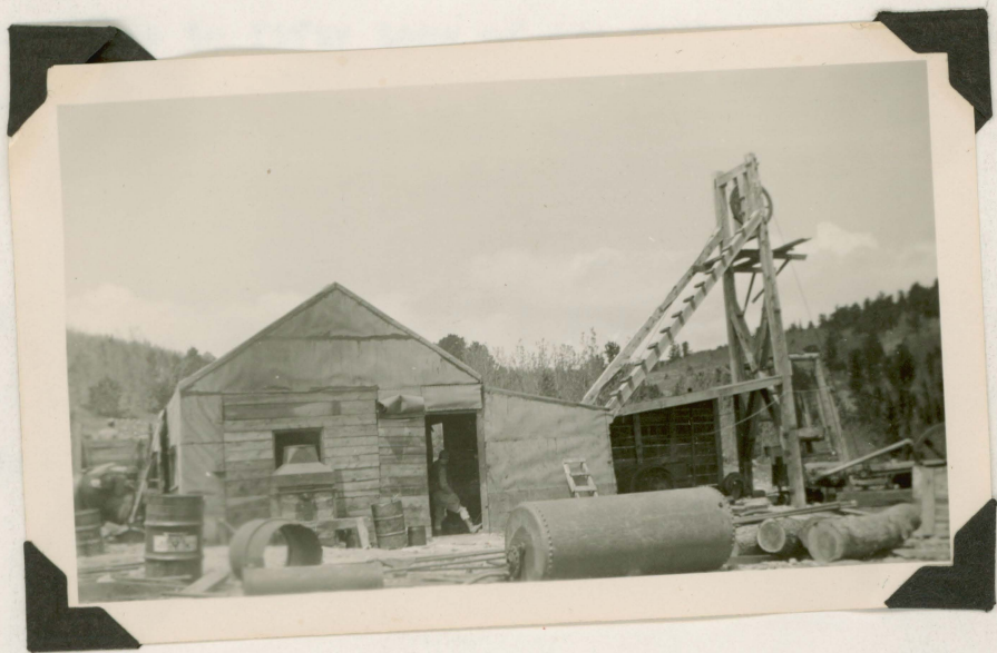
Fig. 5. Shaft house and gallows frame at the Columbia shaft.
