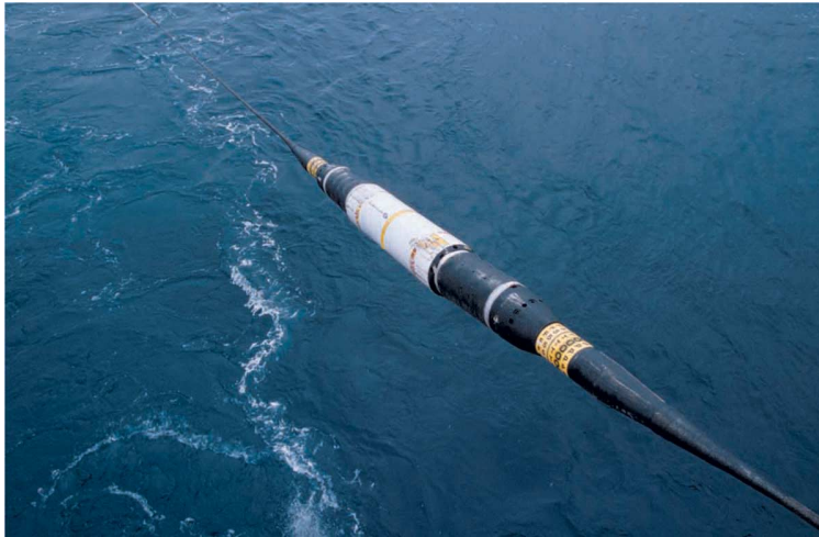
Figure 1.6: An Alcatel Submarine Networks optical repeater being deployed in the ocean. EDFA technology revolutionized global telecommunications in the 1980s and 1990s. The 976 nm, 950 mW fiber Bragg grating stabilized laser diodes used to pump the EDFAs described in Chapter 3 are qualified to the highest Telcordia reliability rating and are certified for use in submarine applications. The front-end laser benefits from the reliability, low cost and availability of fiber-optic components in the 1.5 \mu\text{m} band - although we still avoid flooding in the lab. Photo from Reference [47].
