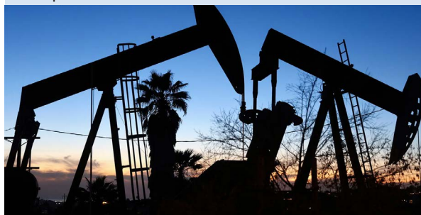
A pumpjack in the Inglewood Oil Field in Los Angeles County, Calif. Photo: Mario Tama/Getty Images.
