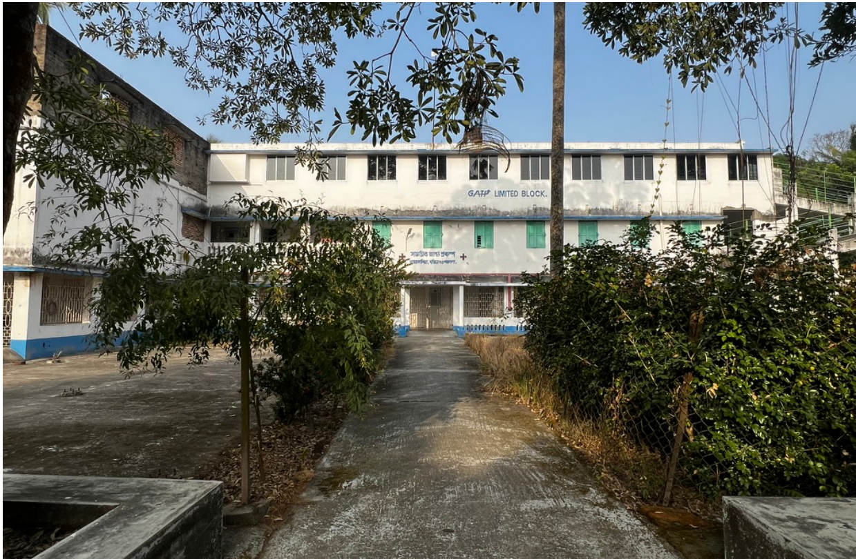
Figure 2: Defunct hospital in Rangabelia village, Gosaba Block, Sundarbans. Photograph taken during preliminary field visit. The image shows an inoperable healthcare facility within the region.
