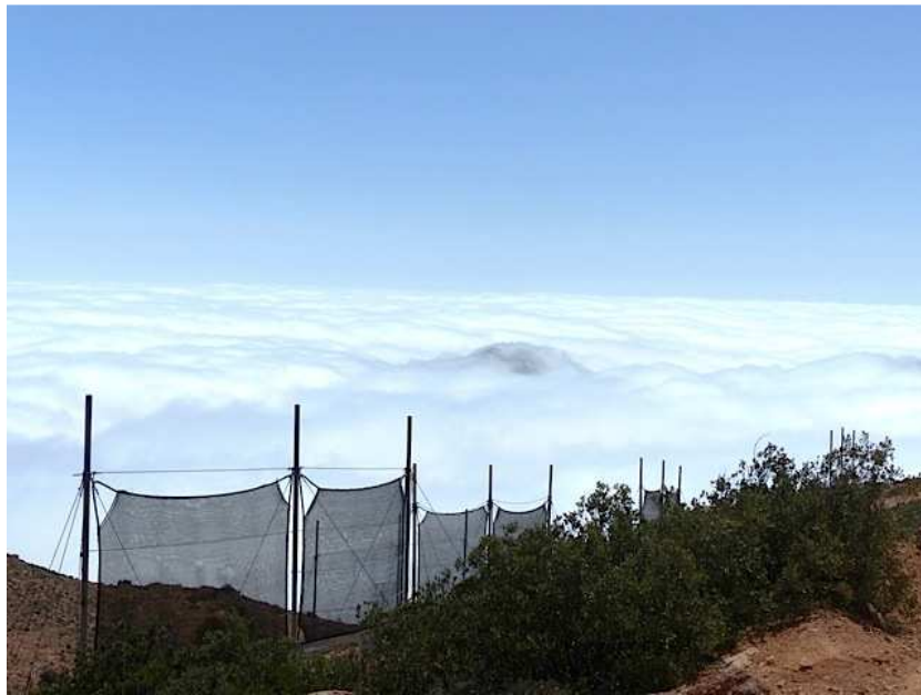
Figure 5: Water-saturated fog clouds and the fogwater harvesting system at the peak of Mt. Boutmezguida.
