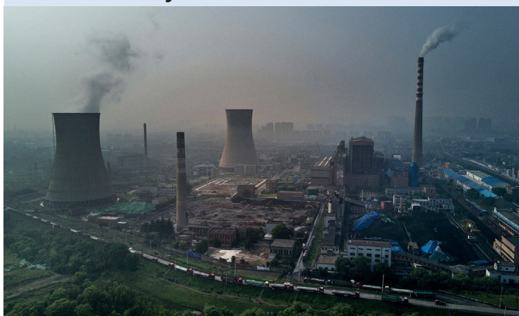
A Chinese state-owned coal-fired power plant is seen near a large floating solar farm project under construction in Huainan, Anhui province, China. Photo: Kevin Frayer/Getty Images.
