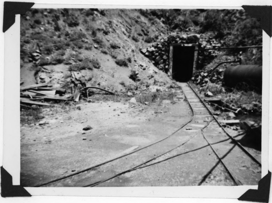
Figure 15. A view of the Portal of Poorman Tunnel
