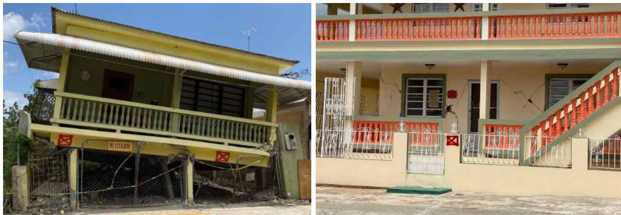
Figure 3.7: Houses in Guánica that were damaged during the January 7, 2020 earthquake. (a) failure in first story columns, (b) shear cracks in masonry walls. [Photos: Polly B. Murray]
