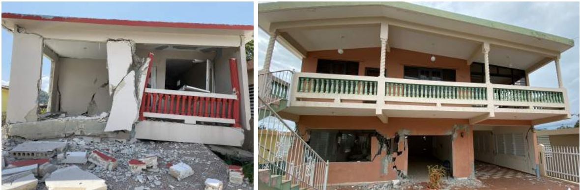
Figure 3.2: Damage to RC houses in Guánica with (a) an open ground story, showing loss of the first open story, and (b) masonry walls between columns at the first story, showing shear cracking in walls and columns. [Photos: Polly B. Murray]
