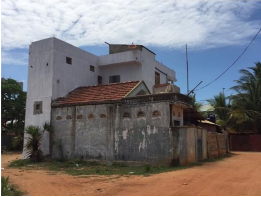
Photo 11: Post-tsunami home with structural additions in New Kattankudy East
