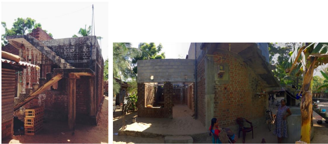
Photo 4: Unfinished homes in Thiruchendur
