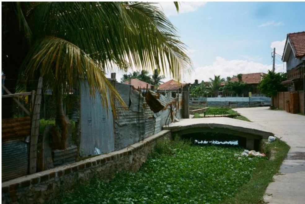
Photo 14: Drainage canal in New Kattankudy East
