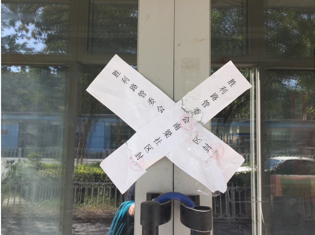
Figure 6.2: The notification of demolition by the shequ . Both of the pieces of paper say the same thing: Victory Road Management Committee Nanliang Shequ Letter: May 2017. Source : Photo by author, May 2017.
