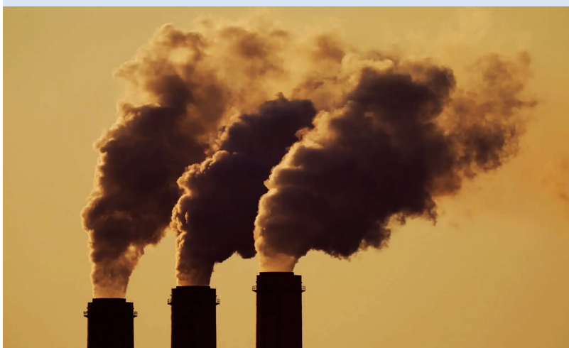
A coal-fired power plant in Kansas in 2021. Photo credit: Charlie Riedel/ Associated Press .
