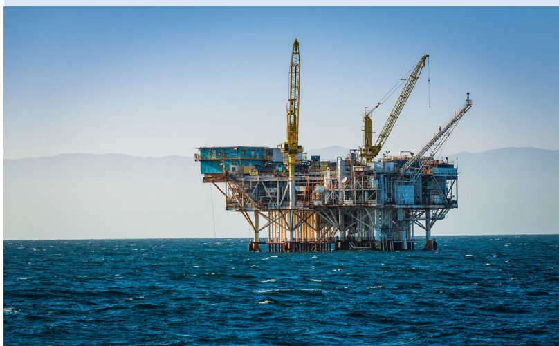
Off-shore oil platform in the Santa Barbara channel, off Ventura, California. Photo credit: Russ Bishop/Alamy.
