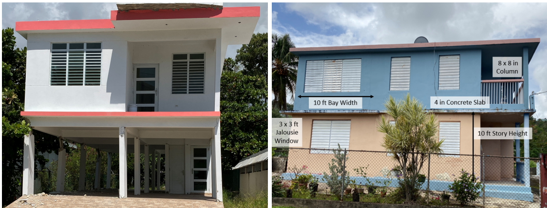
Figure 3.5: Typical RC houses in Guánica and Humacao, Puerto Rico. [Photos: Polly B. Murray]
