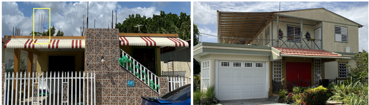
Figure 3.3: (a) Puerto Rican home with exposed reinforcing bars to facilitate house expansion. (b) Home with RC first story and wood frame second story (Yabucoa, Puerto Rico)[Photos: Polly B. Murray]
