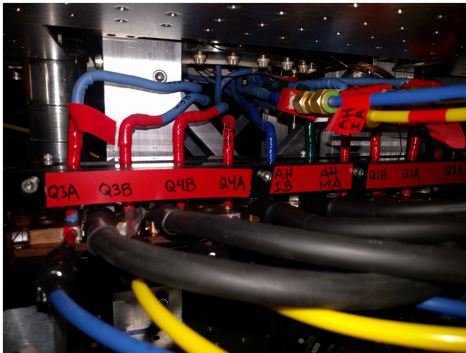
Figure 2.28: Top: CAD model of the water and electrical hookups for the bottom bucket coils. Bottom: Photo of the connections under the main chamber.
