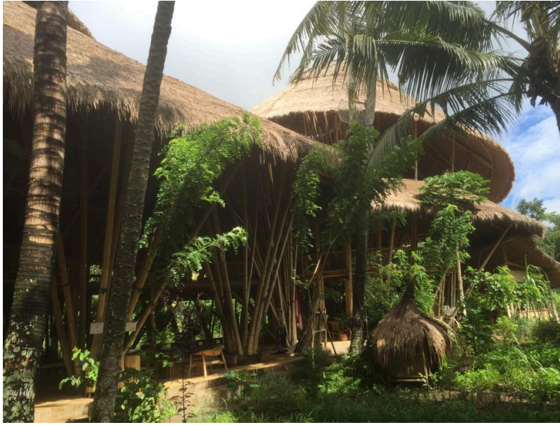
Figure 7 The Green School in Bali. Credit: Lawrence Flynn
