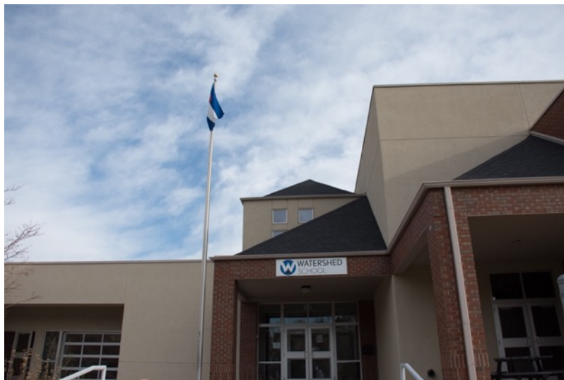
Figure 23 Watershed School. Central Boulder, Colorado
