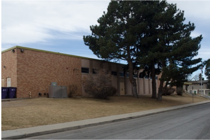
Figure 29 Denver Green School. Glendale neighborhood of Denver, Colorado
