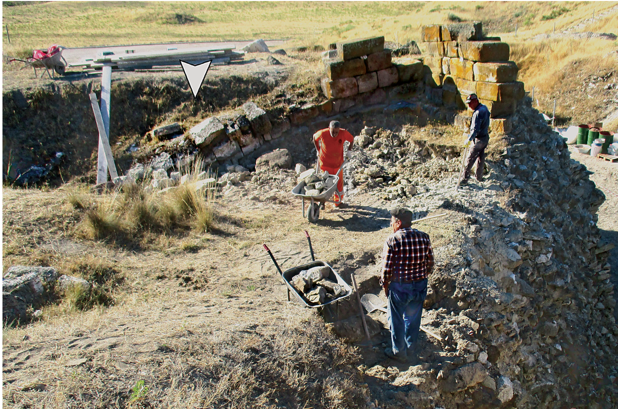
Fig 30. Interior face of the southeast corner of the North Court of the Middle Phrygian Gate Complex, showing significant subsidence before collapse (i.e., in the wall sloping down to the left at the rear of the image [marked by a white arrow]). The wall was the interior face of the north-south wall on the eastern edge of the Middle Phrygian Gate Complex's North Court. This wall was originally horizontal before subsidence in antiquity. (Photo by S. Gönen)
