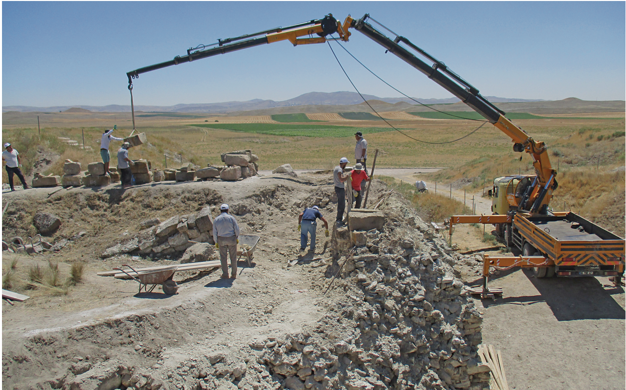
Fig. 24. Removing stones with a mobile crane. (Photo by S. Gönen)
