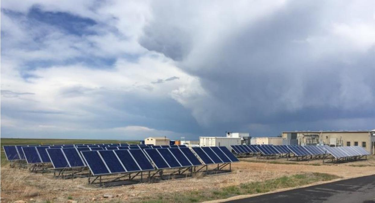
**Figure 17. The two identical PV arrays used for experimental validation of MPPE and RAPC. One array is in the left foreground, and the second is to the right and slightly behind it. The inverter and test equipment are located in the DERTF building behind the right hand array.**
